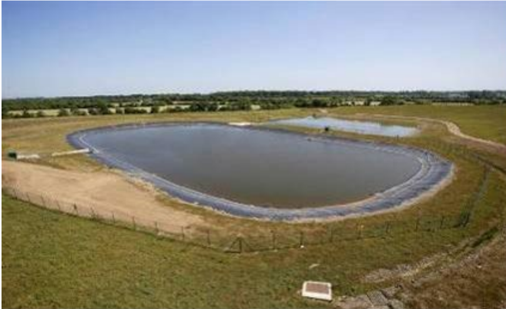
Plate 1-5: Surface Water Attenuation Pond and Wetland
