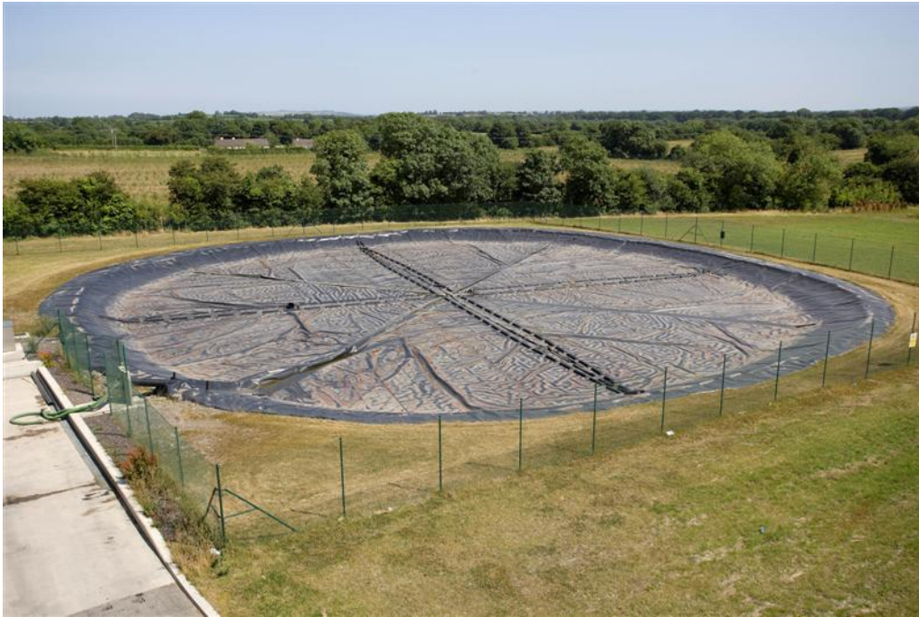
Plate 1-4: Covered Leachate Lagoon
