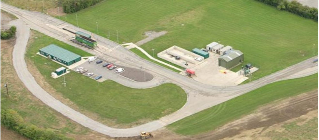
Plate 1-2: Knockharley Landfill Administration Area
